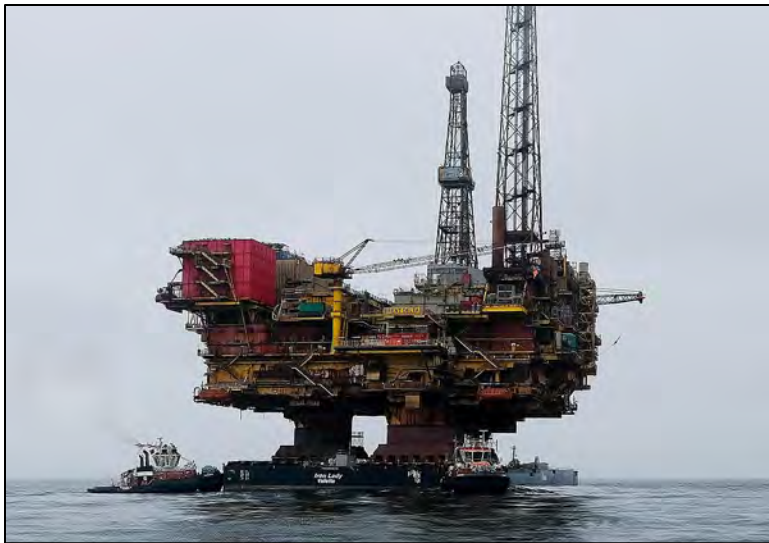
Figure 15. Iron Lady barge transporting the Brent Delta topside (Shell 2017b)
