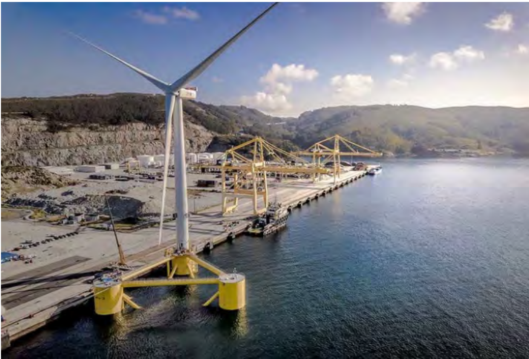
FIGURE 4-2: WTG COMPONENTS ASSEMBLED ON SEMI-SUBMERSIBLE FOUNDATION AT QUAYSIDE (Source: Principle Power)
