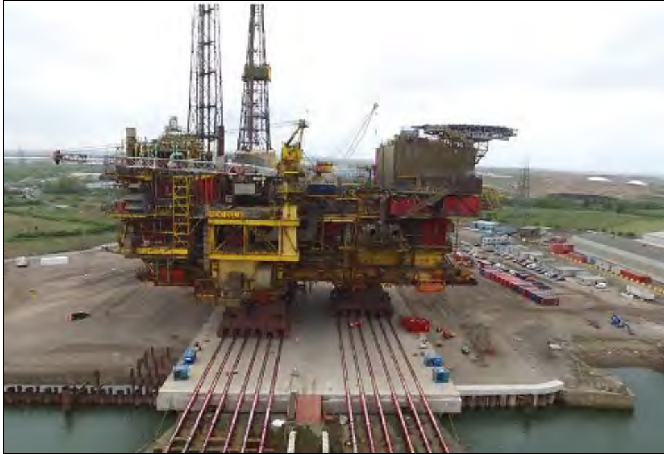
Figure 17. Skidding Brent Delta topside onto Able Seaton Port (Shell 2019)
