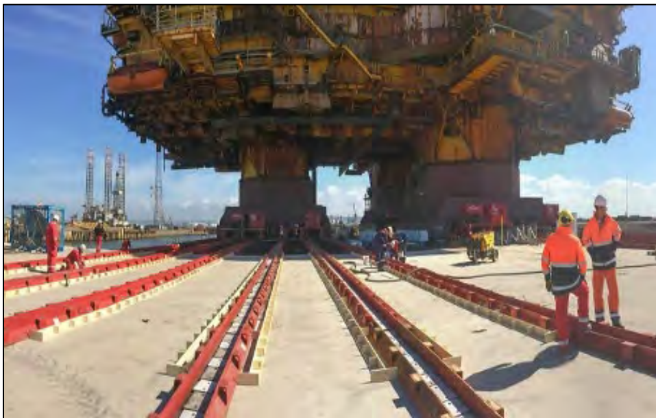
Figure 18. Skidding Brent Delta topside onto Able Seaton Port (Shell 2019)
