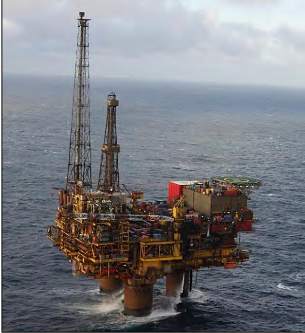
Figure 13. Photo of Brent Delta prior to decommissioning in the North Sea (Adams 2015)
