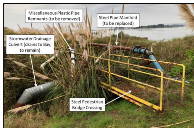
Image 1: Existing stormwater feature to be replaced
