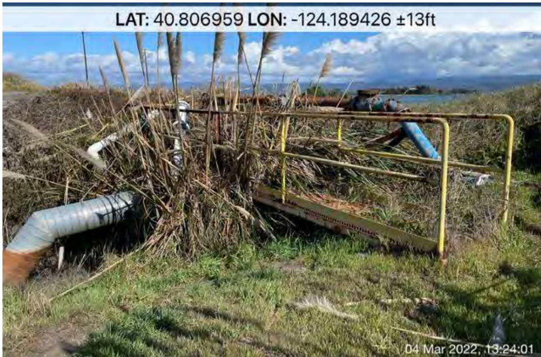
Photo 7: Existing stormwater detention facilities looking northeast. ESHA is not present at this location. Pipeline and bridge alignment would likely pass over here. Photo taken March 4, 2022.
