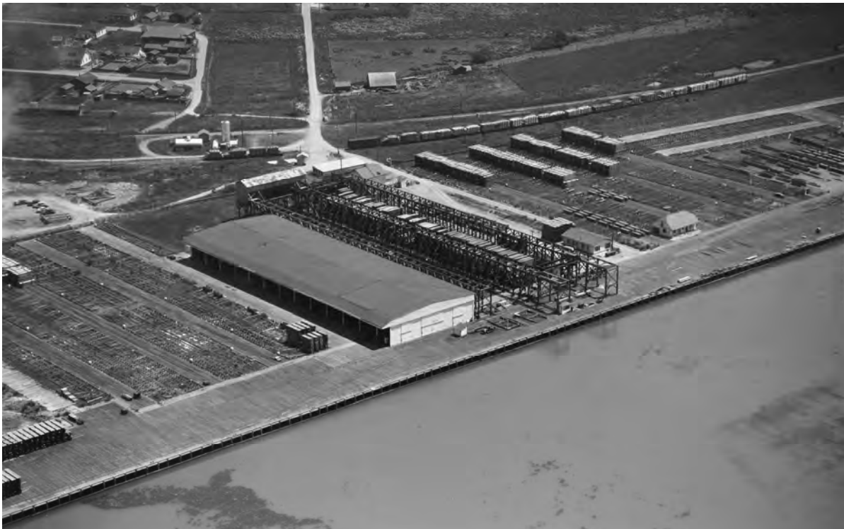
Figure 1. 1947 aerial photo showing former Kramer Dock and supporting piles (Humboldt Room 1947).
