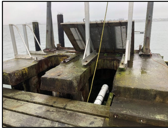
Image 5: Existing concrete sea-chest and screens at the Red Tank Dock. This sea chest will continue to be utilized; the screens will be replaced.
