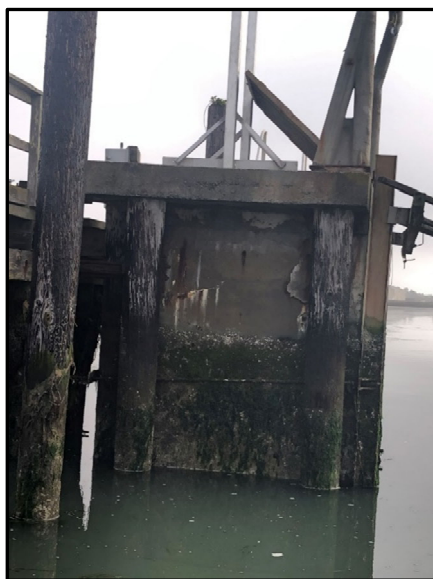
Image 6: Existing concrete sea-chest at the Red Tank Dock. This sea chest will continue to be utilized.
