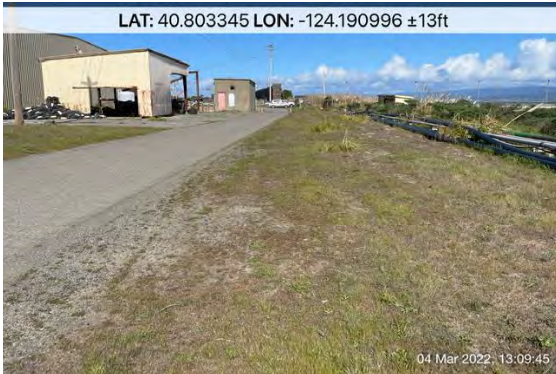
Photo 4: Southern pipe alignment looking north. Compacted gravel soils. Photo taken March 4, 2022.
