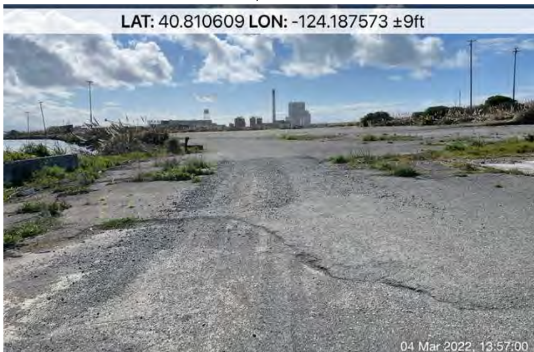
Photo 10: Typical conditions throughout the majority of the pipeline alignment. Note expansive areas of asphalt. Photo looking south taken on March 4, 2022.
