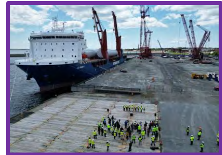
Figure 1 Loading Steel Towers
