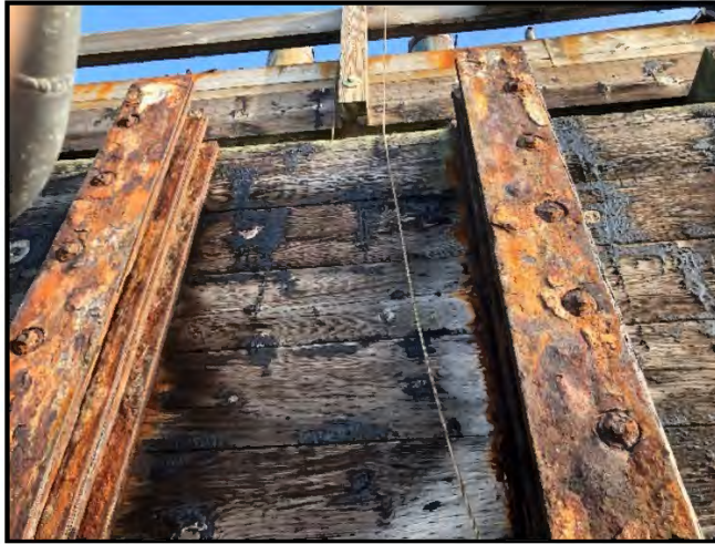
Image 3: Existing wooden sea chest at the Redwood Marine Terminal II Dock.
