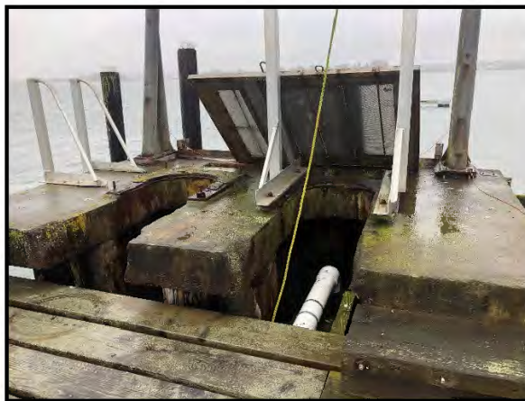
Image 5: Existing concrete sea-chest and screens at the Red Tank Dock.
