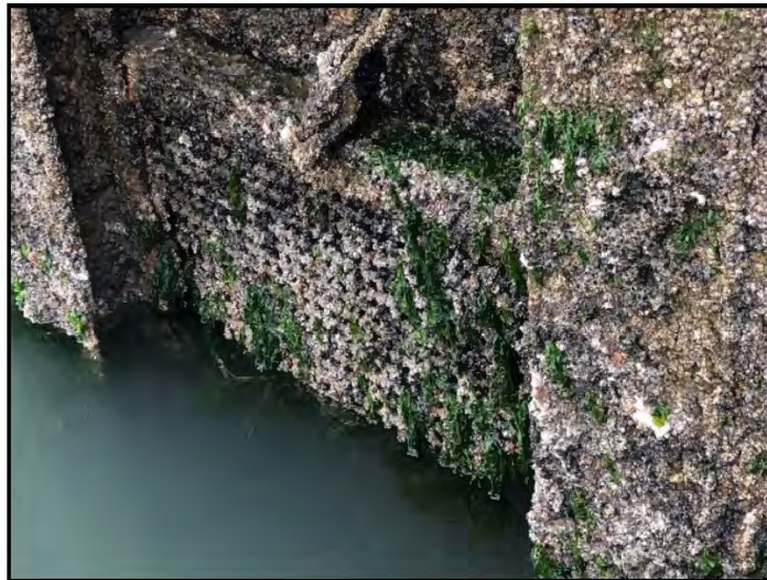
Image 4: Existing water intake screen at the Redwood Marine Terminal II Dock.
