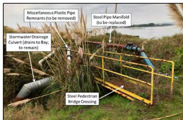
Image 1: Existing stormwater feature to be replaced
