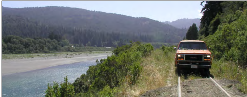
Figure 3. Section of the NCRA Railroad in the Eel River Canyon
