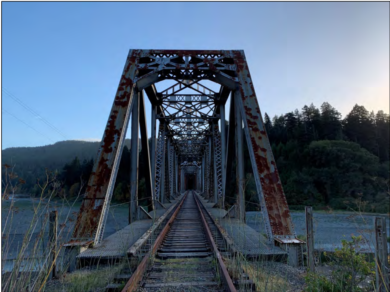
Figure 5. Aging Railroad Trestle in NCRA Corridor
