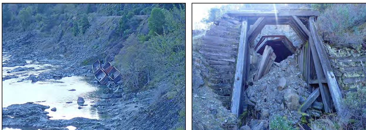
Figure 18. Rail Cars and Collapsed Tunnel in Eel River Canyon
