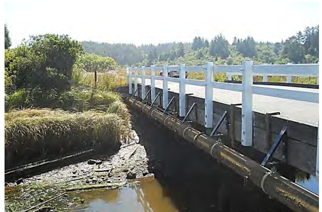
Figure 3: Existing Water Line
