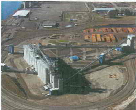
Figure 11 – EGT Longview Terminal
